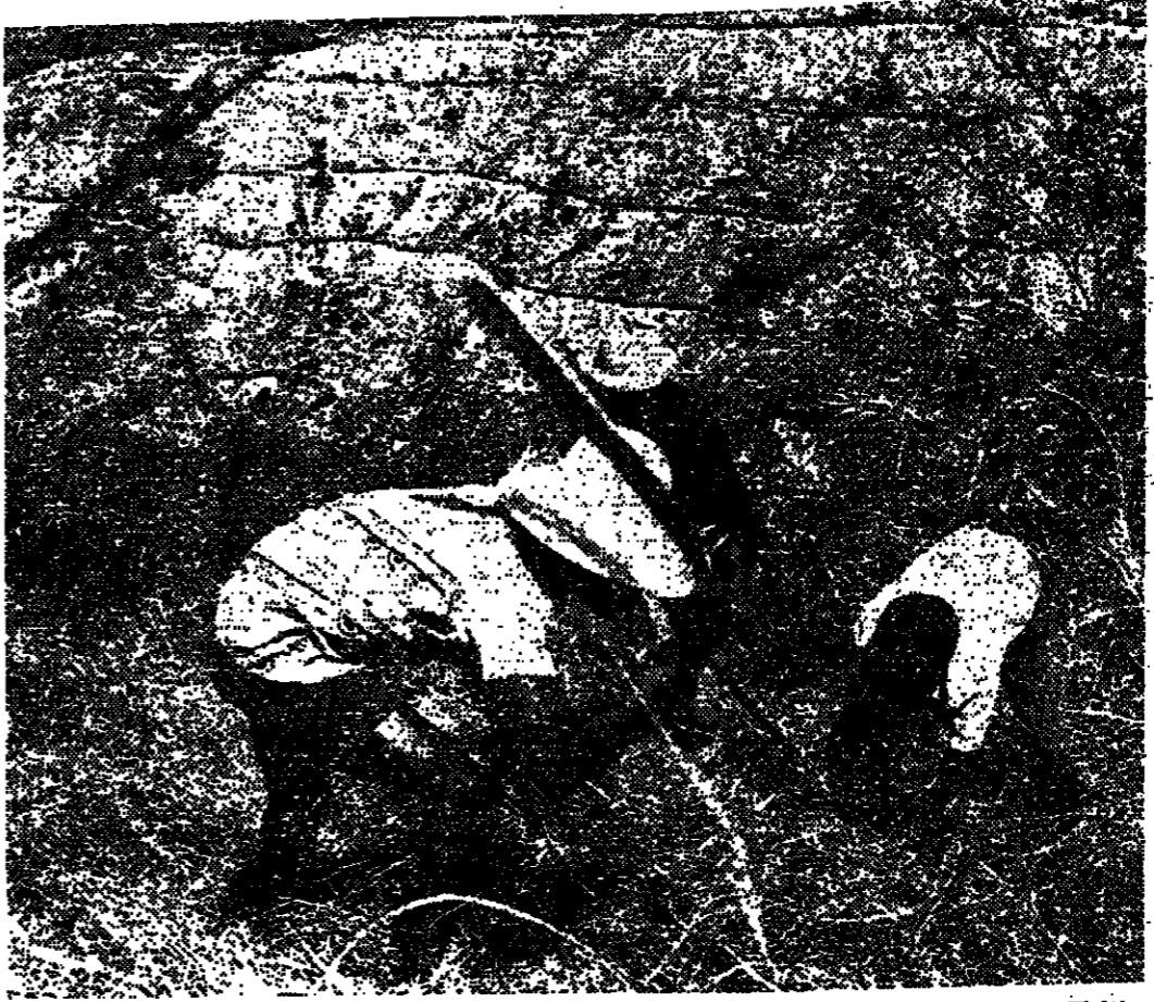
Clearing hillside undergrowth for terracing—part of the "food for work" project in Haiti.
